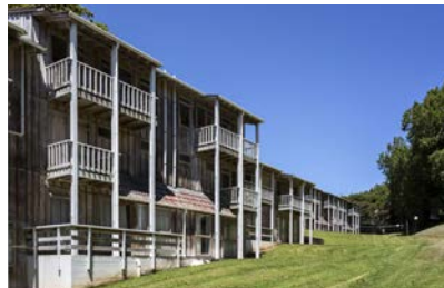
Parnell Student Village 8 Claybrook Road, Parnell, Auckland
